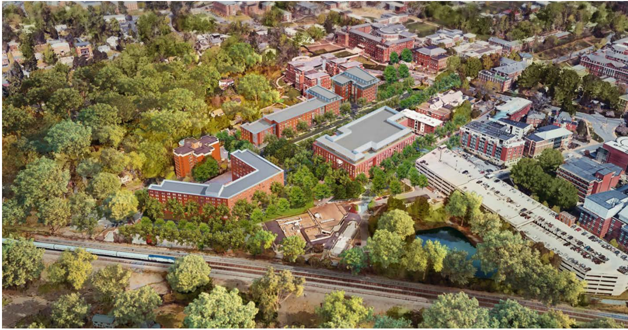
Aerial View Looking North
