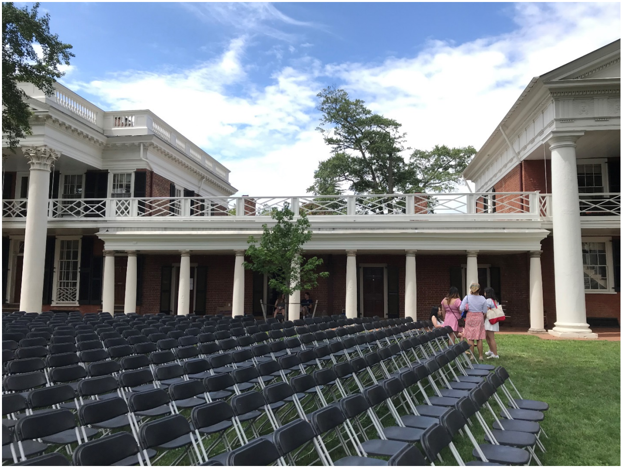
New railing seen from the Lawn. Also note the restored Colonnade columns with their final paint coat.
