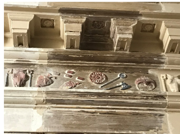
Paint removal test on parlor cornice
