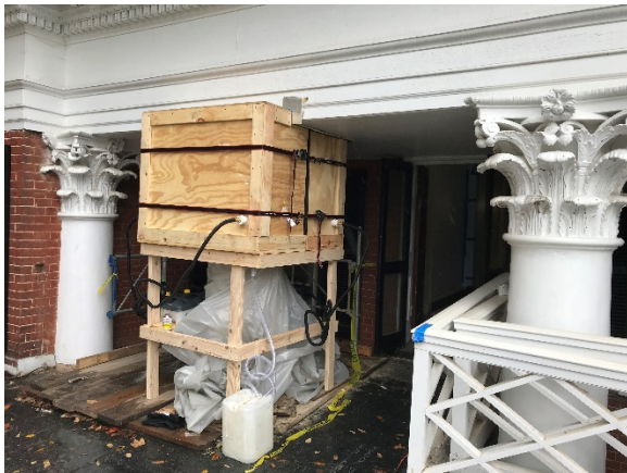
Steam box used to remove paint
