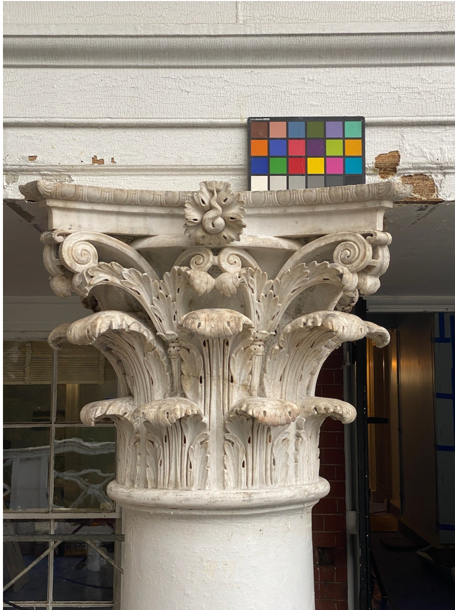
Original capital at Pavilion VIII after paint removal
