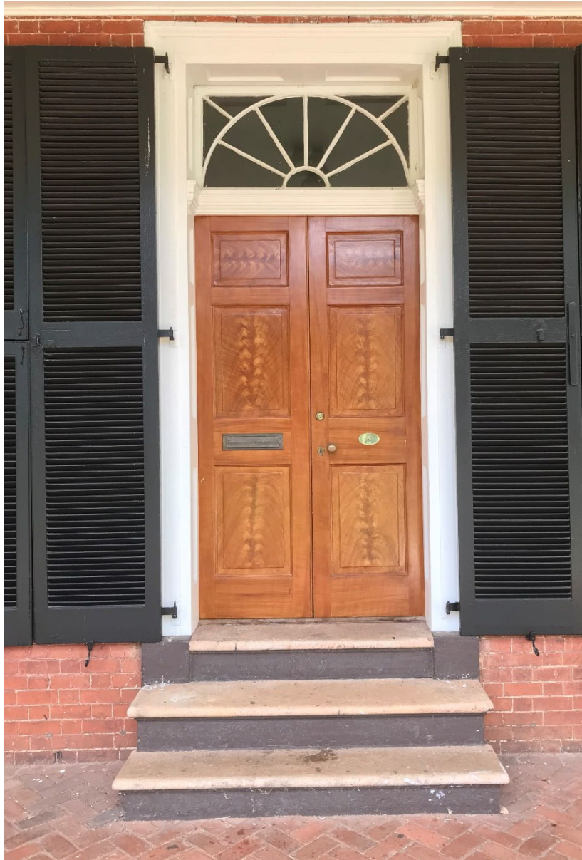
Recently grained door at Pavilion V
