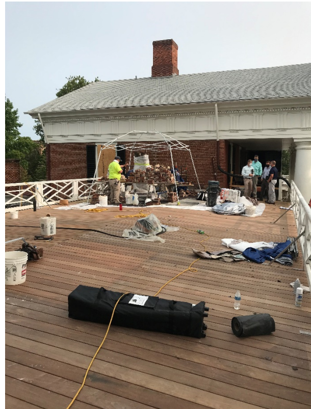
New roof & chimney repair near completion
