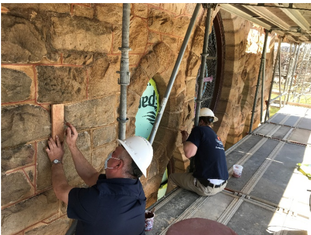
Repointing Chapel façade
