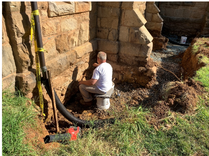
Below-grade masonry repairs
