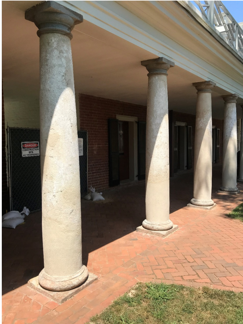
Restored columns awaiting the paint coat on their shafts
