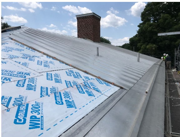
New roof being installed
