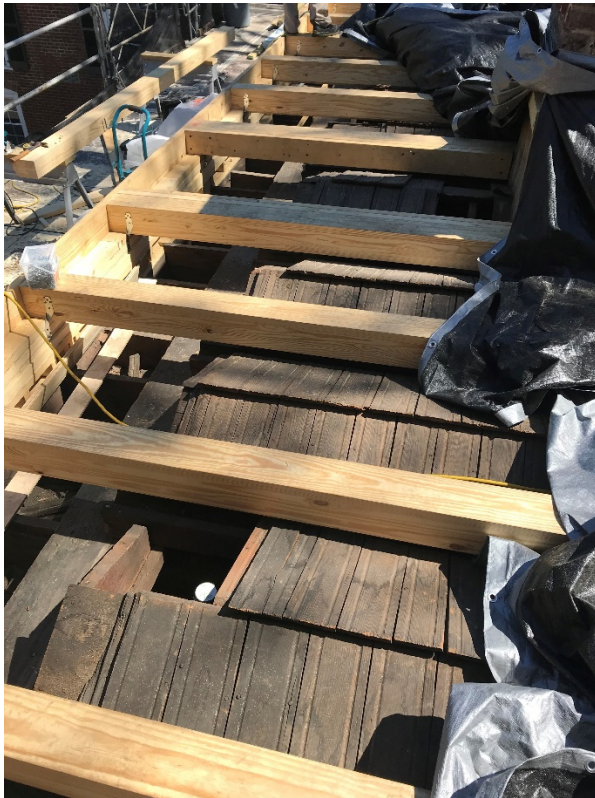
Sections of original roof being encapsulated by new roof structure
