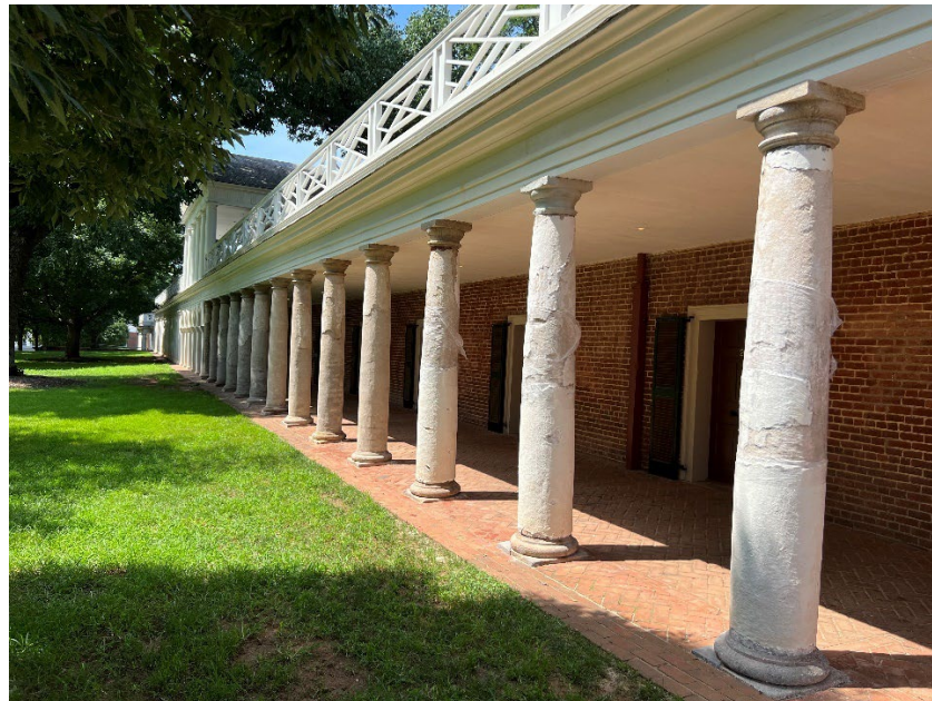
Columns being restored south of Pavilion V
