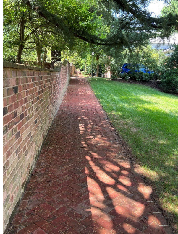
New brick walk at Pavilion III
