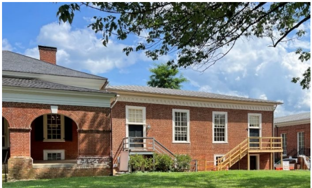
New stair under construction
