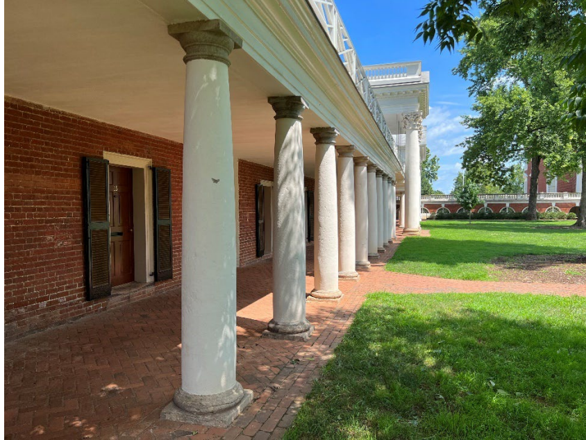
Completed columns south of Pavilion III
