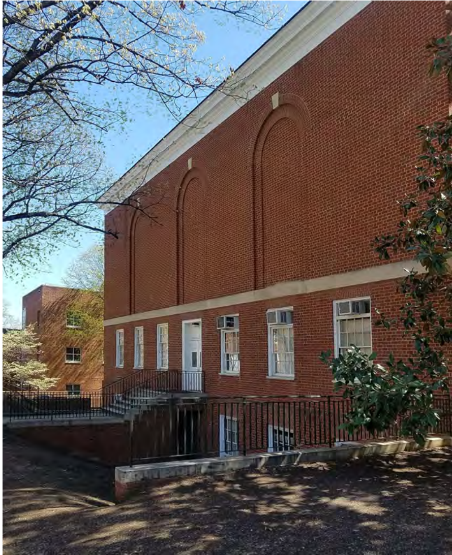
Existing West Facade
