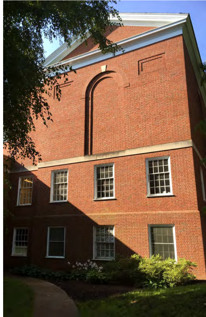
Existing North Facade
