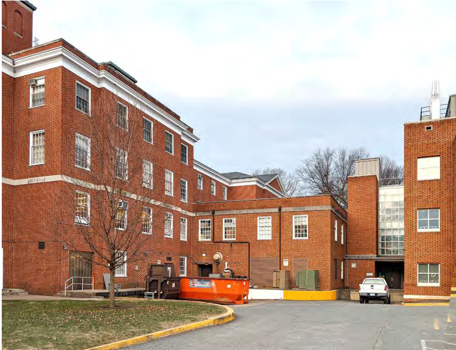
Current view from parking area and loading dock
