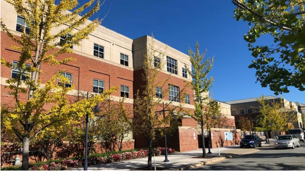
Existing northwest view of the UVA Encompass Health Rehabilitation Hospital
