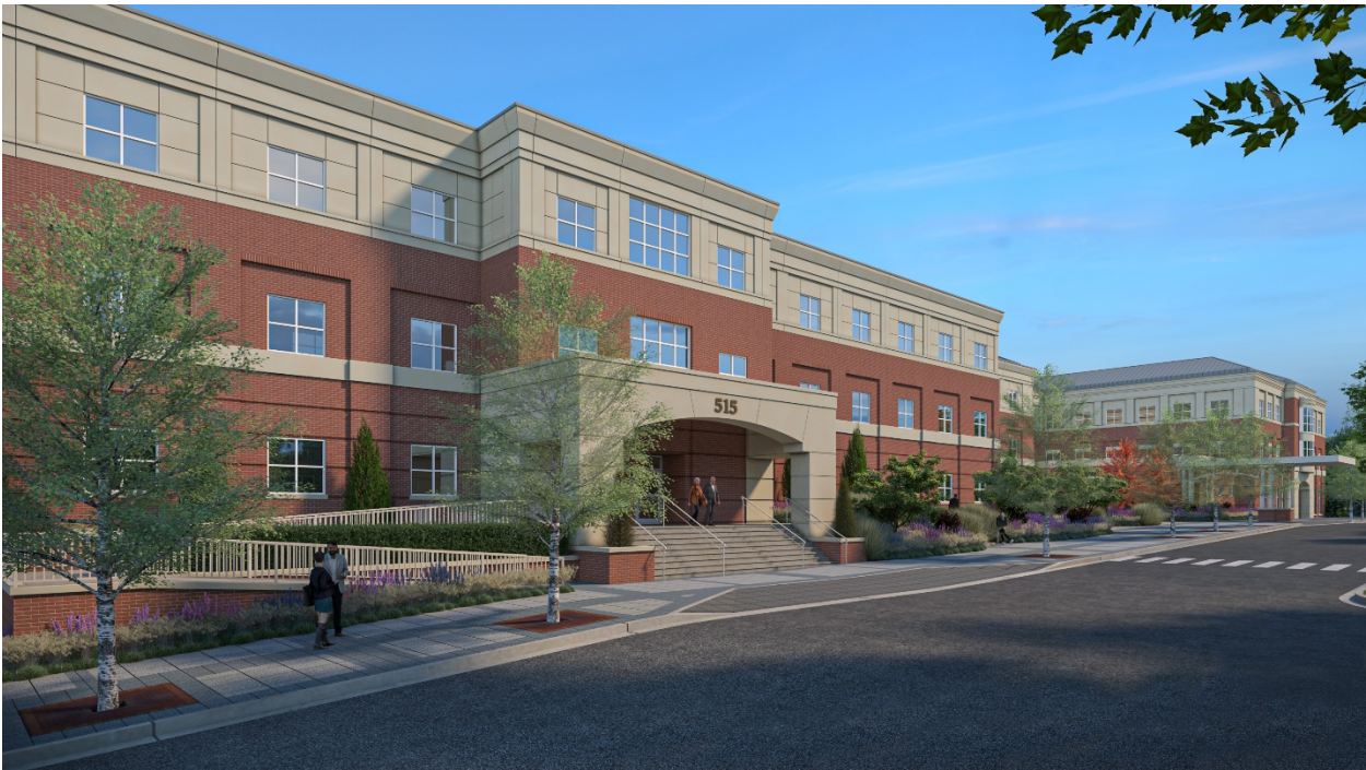
Proposed northwest view of the UVA Encompass Health Rehabilitation Hospital, showing new stairs, accessible ramp, and two-story addition
