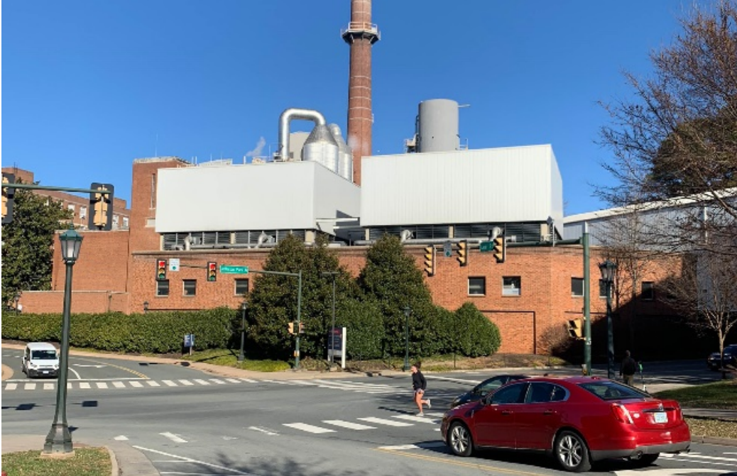
Existing View of Plant from Lee Street
