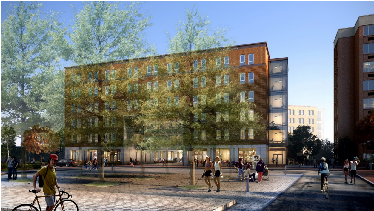
New Upper Class Student Housing (under construction)
