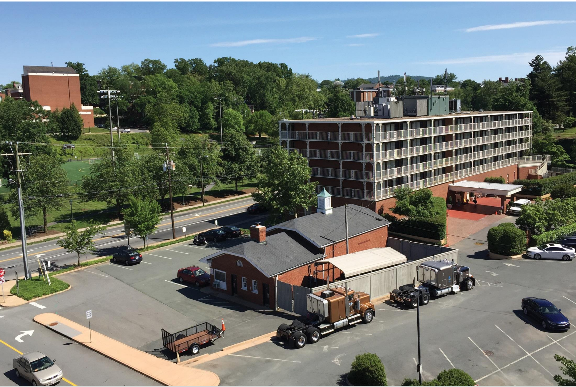
Existing view from parking Garage (looking east)
