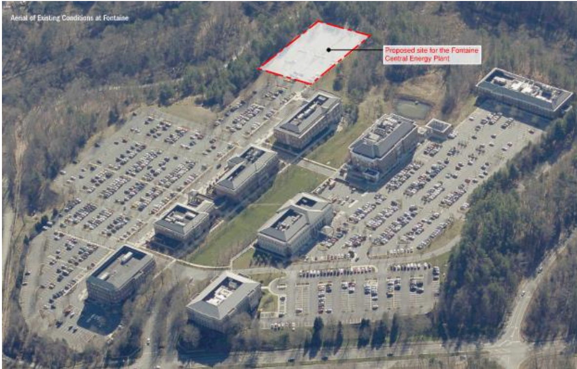
Existing conditions at Fontaine Research Park with proposed site for the CEP
