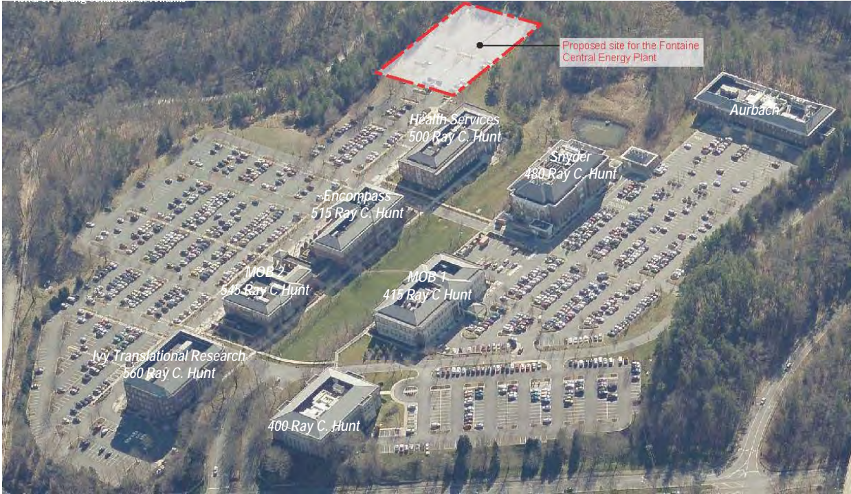
Existing conditions at Fontaine Park with approved site for the Central Energy Plant
