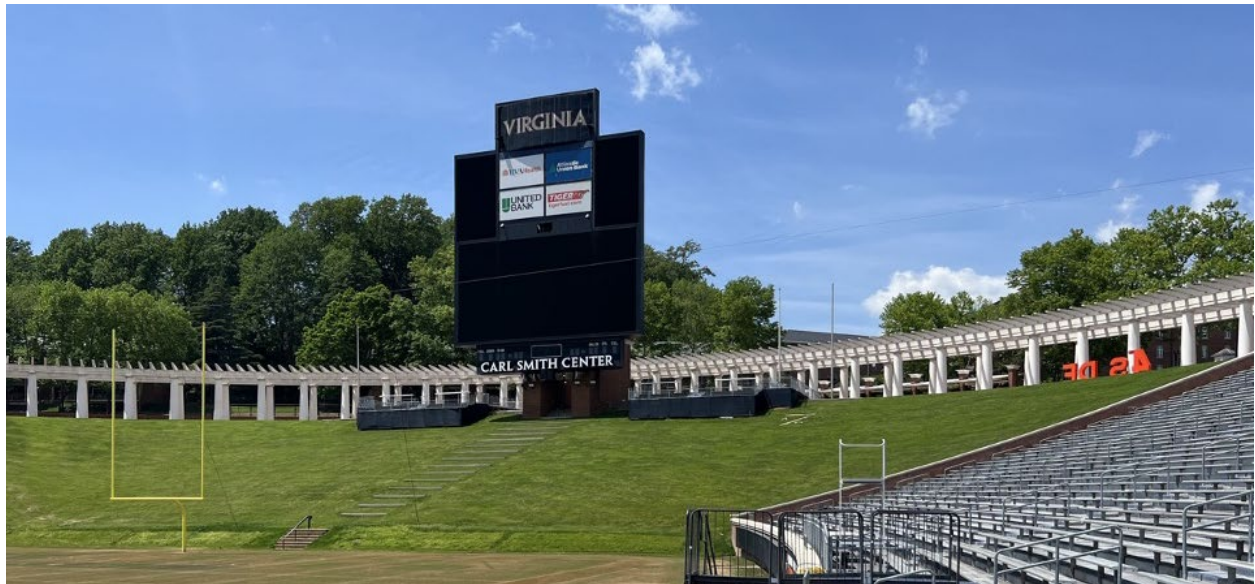
Existing Scott Stadium Video Scoreboard – Field View
