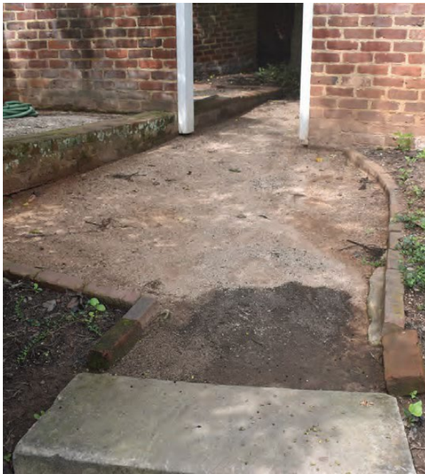
Garden II paving, before
