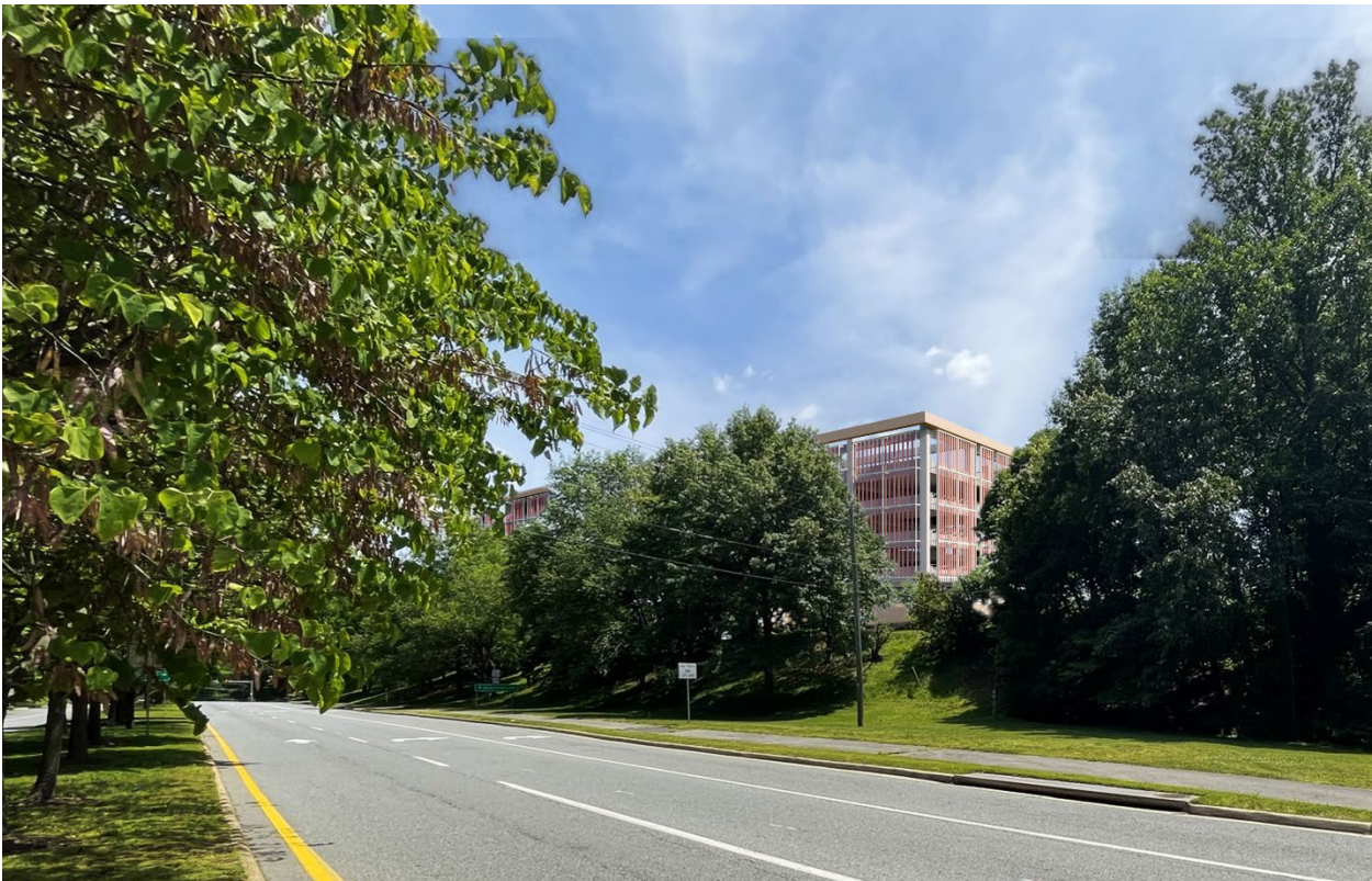
View of Parking Garage from Fontaine Avenue
