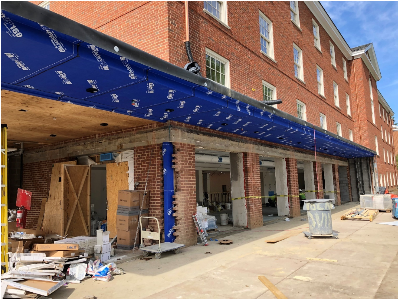
Figure 2: McCormick Road Residence Halls (here, Bonnycastle) under construction
