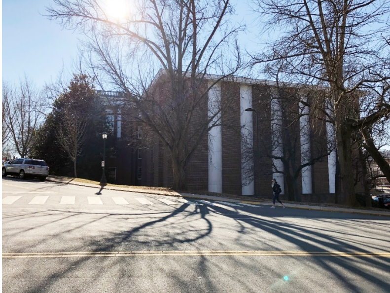
Present-day view of existing portion of building to be demolished
