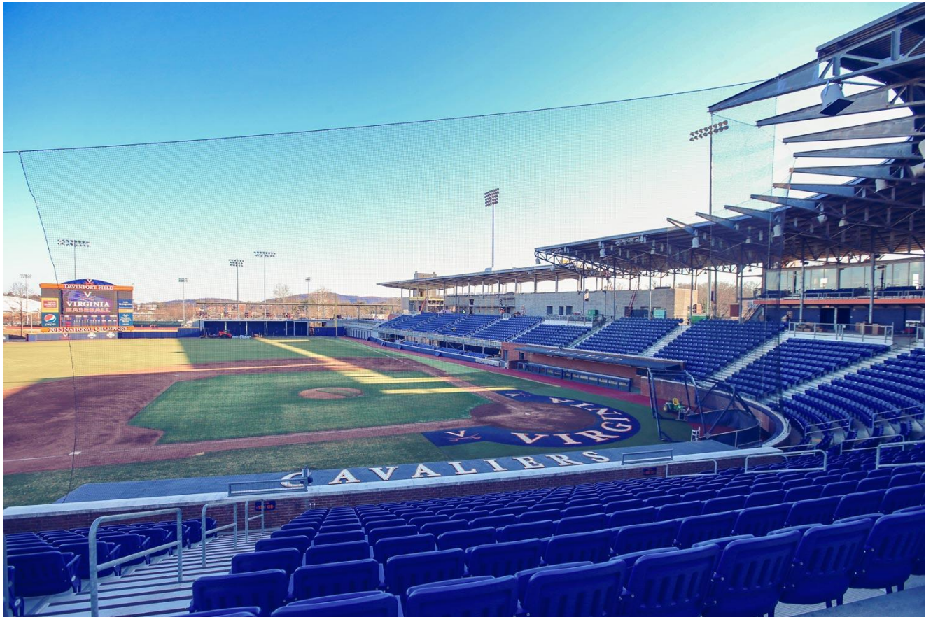
Figure 3: Davenport Stadium was one of many projects receiving occupancy this fiscal year
