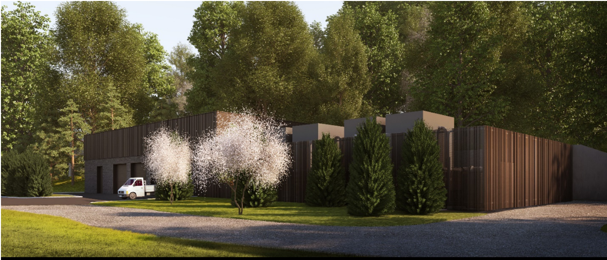
Central Utility Plant West Perspective
