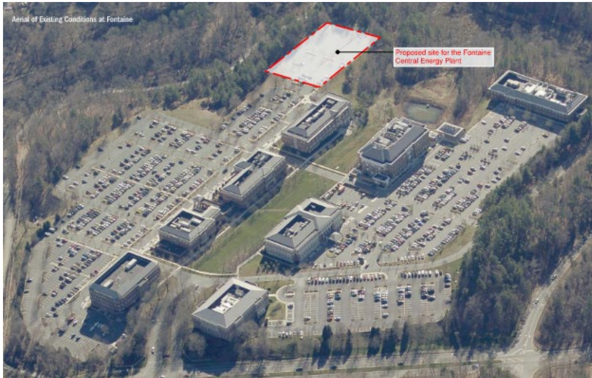
Existing conditions at Fontaine Park with proposed site for the FCEP
