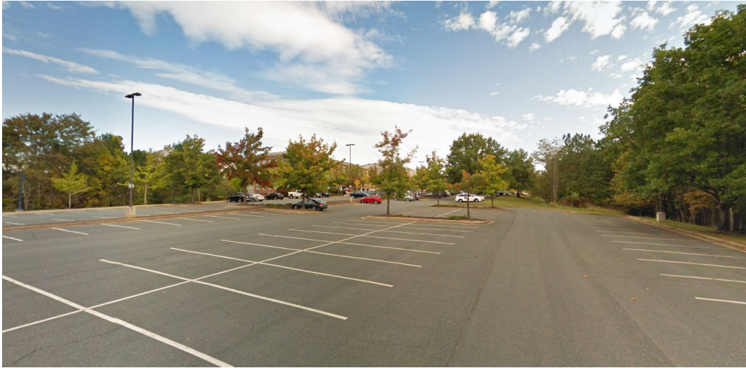
Existing conditions at proposed site for the Fontaine Central Energy Plant
