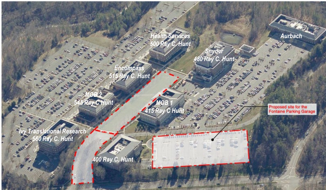
Existing conditions at Fontaine Park with proposed site for roadway Infrastructure & Parking Garage
