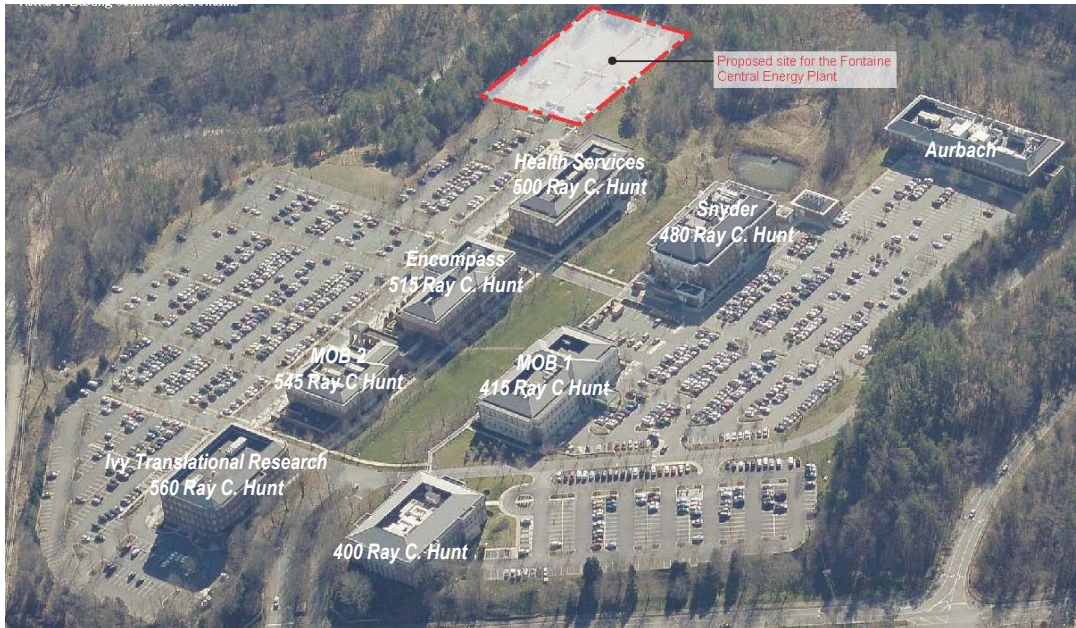
Existing conditions at Fontaine Park with proposed site for the Fontaine Central Energy Plant
