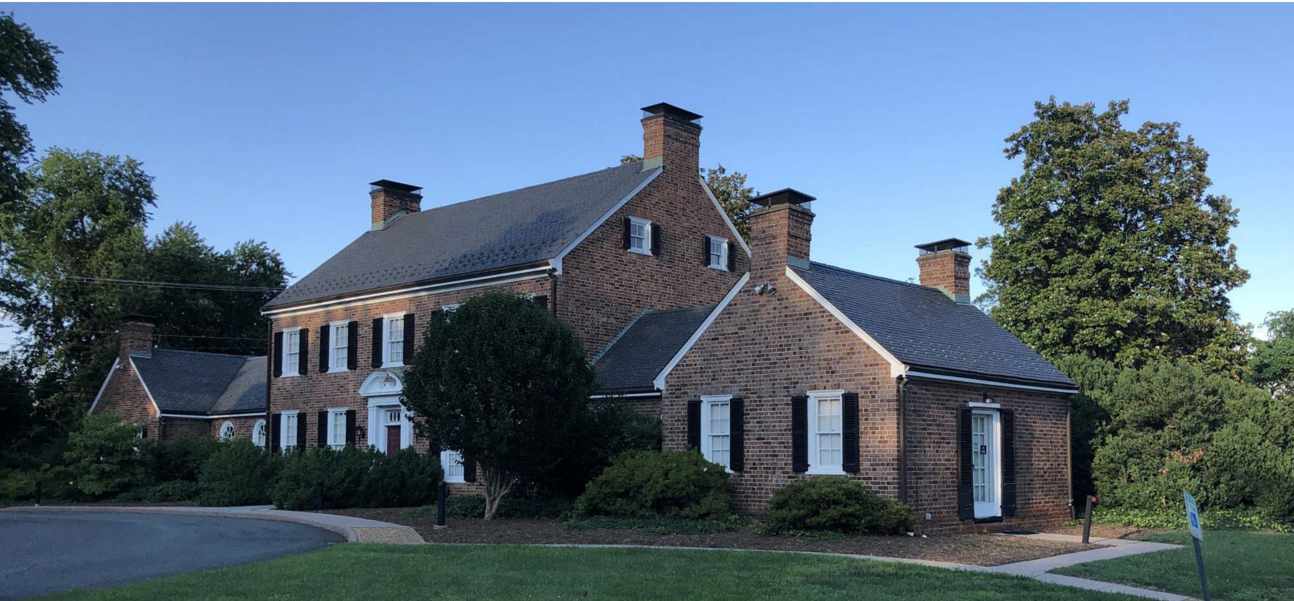
Existing View of Montesano, Looking Northeast
