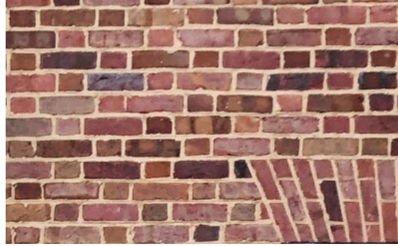
Brick Matching Existing House
