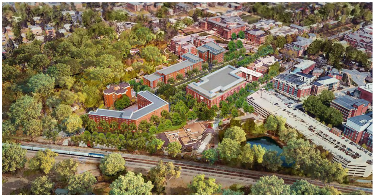
Aerial View Looking North
