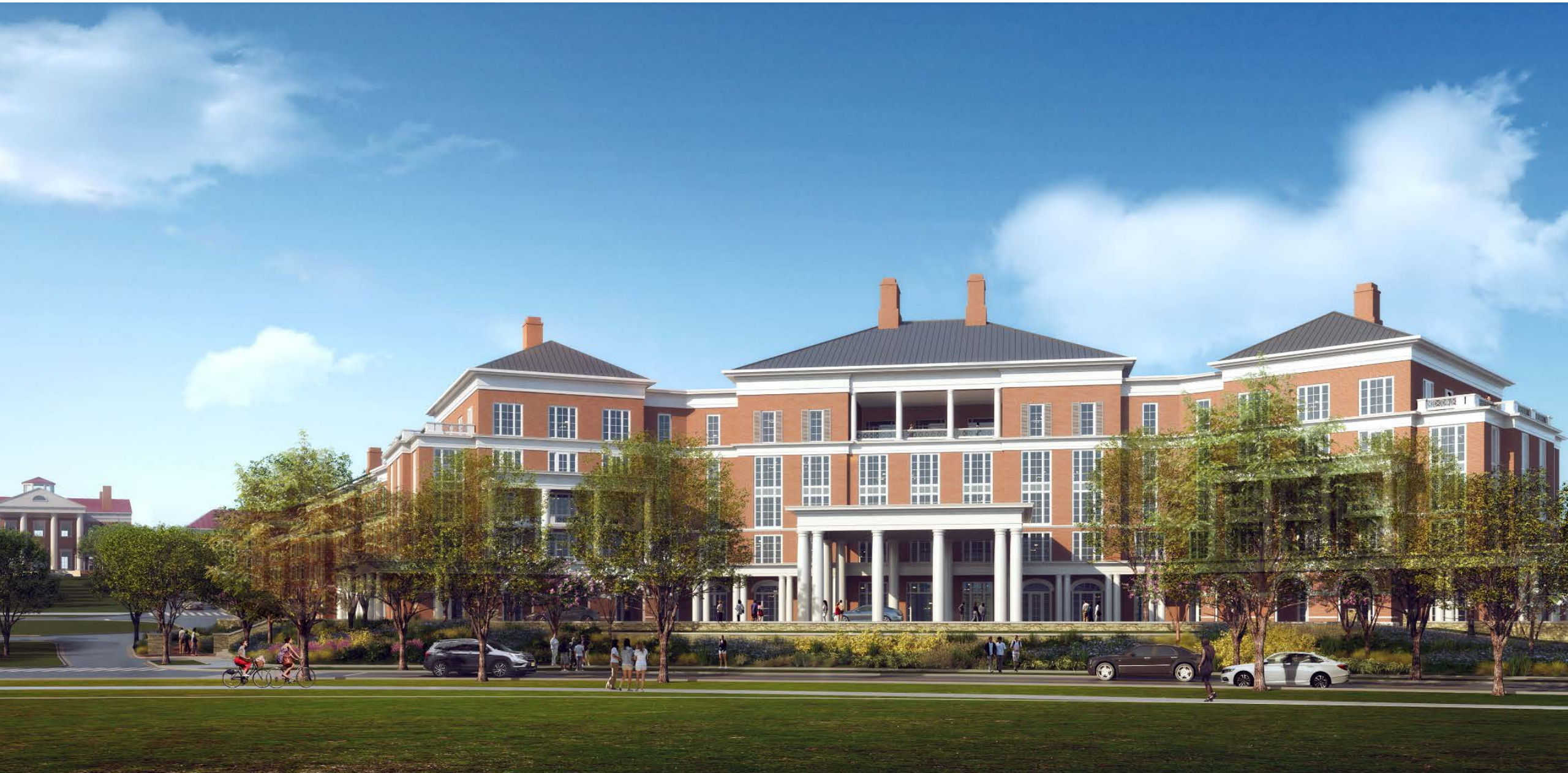
Proposed view of the Inn at Darden, looking north toward Saunders Hall
