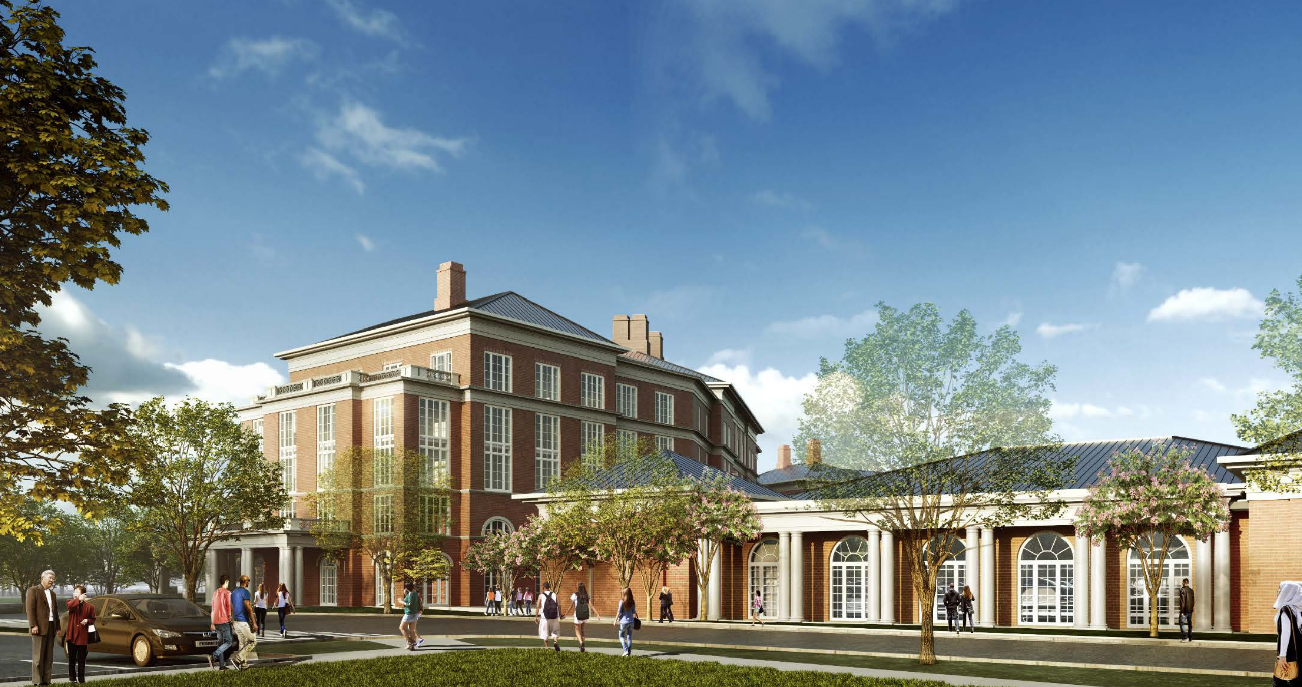
Proposed view of the Inn at Darden, looking west toward the conference center
