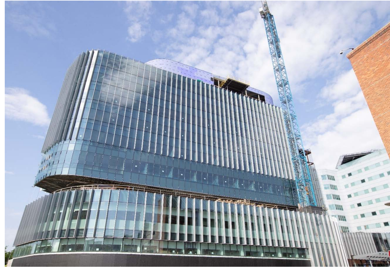
University Hospital Expansion project under construction
