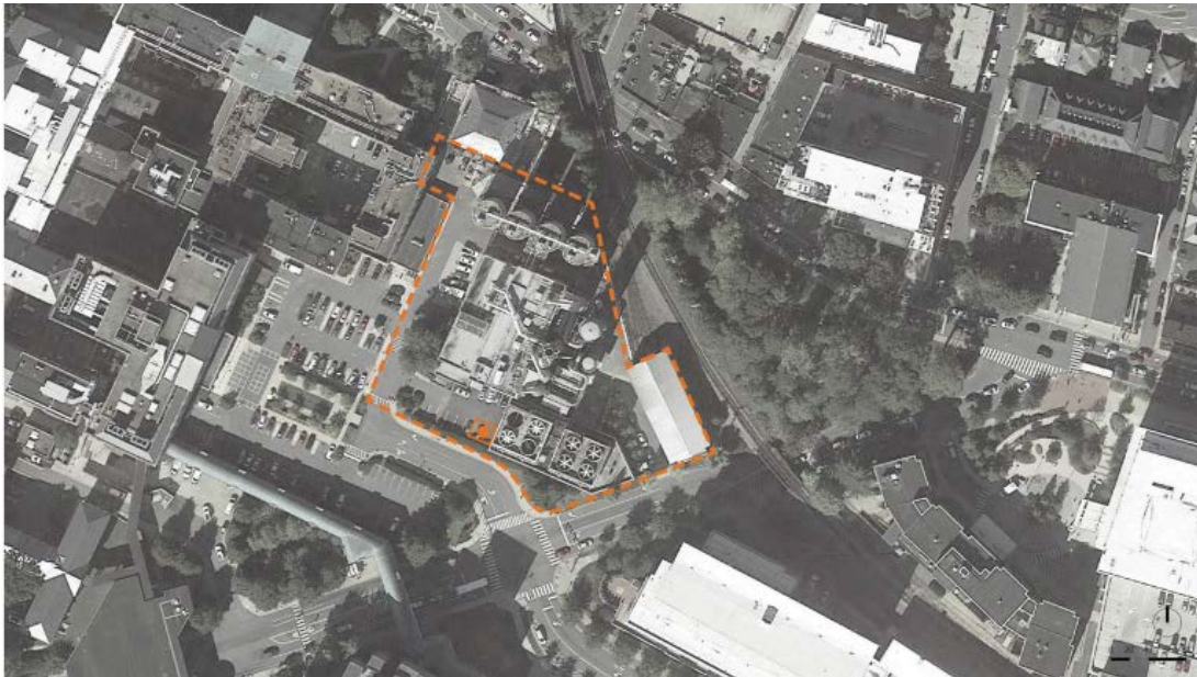
Location of North Chiller Plant on Jefferson Park Avenue and Lee Street
