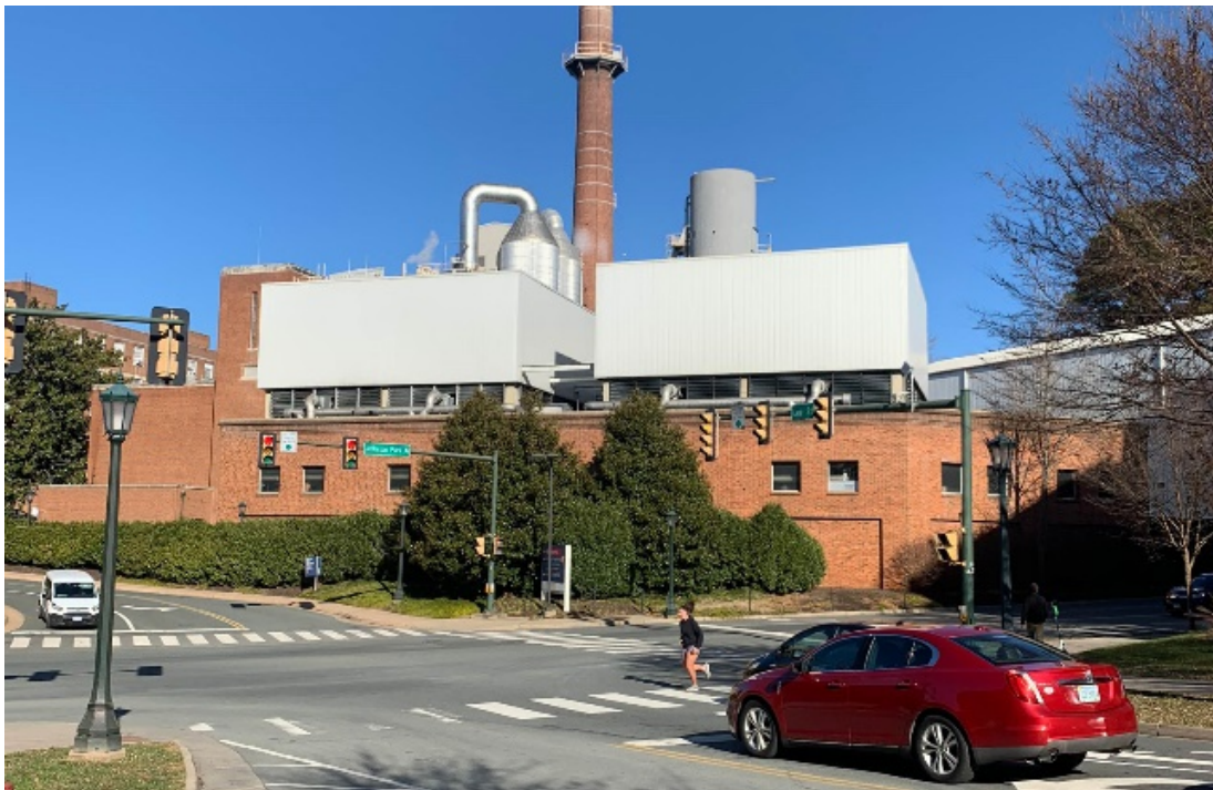
Existing View of Plant from Lee Street
