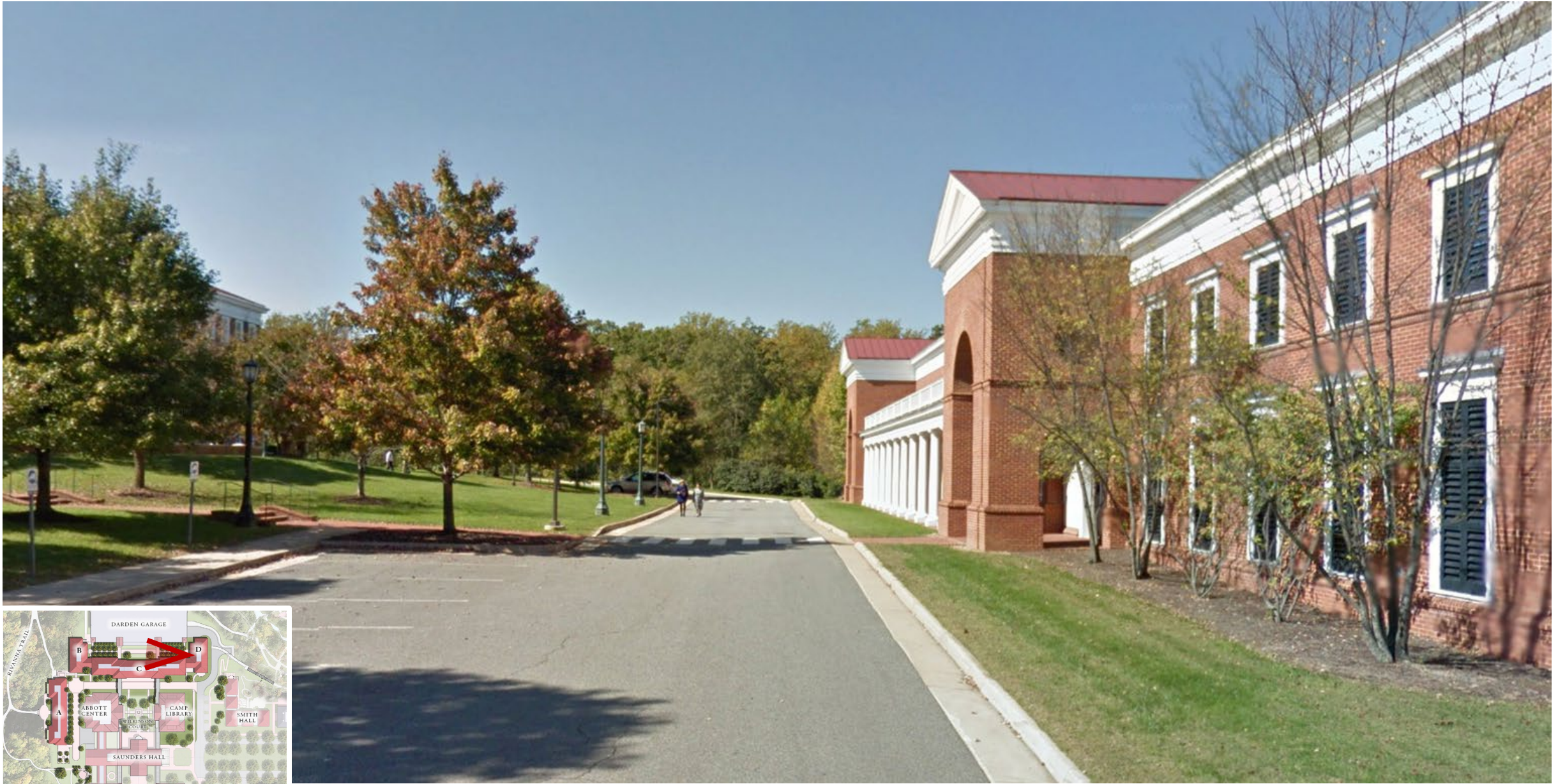
VIEW OF BUILDING B FROM NEW COURT – EXISTING
