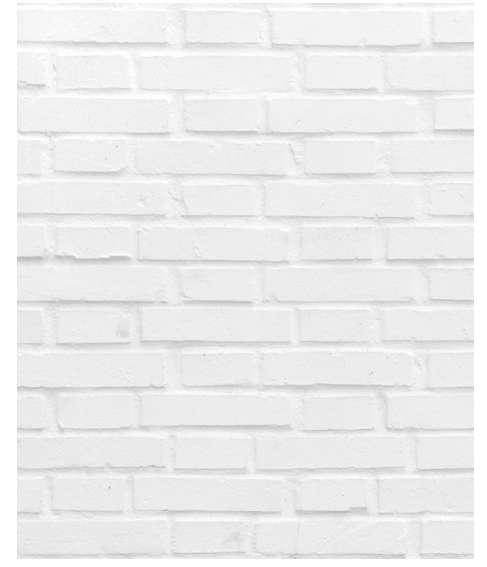
PAINTED BRICK – NICHES & BREEZEWAY WALLS
