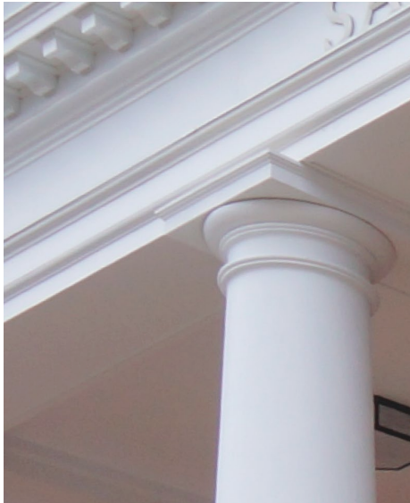
FIBERGLASS – CORNICES, SPANDRELS
