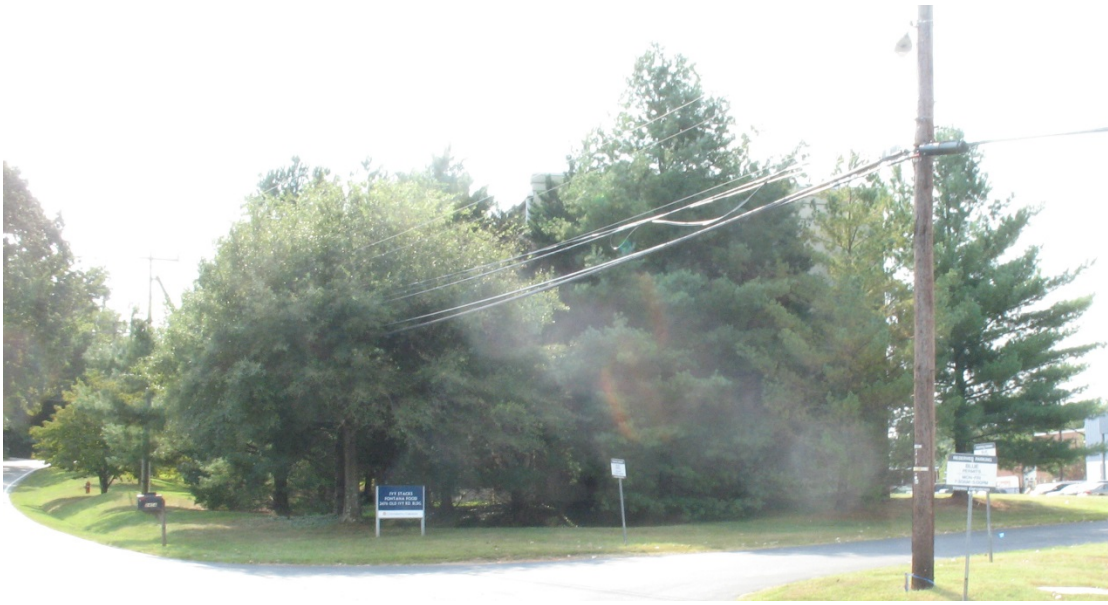
View of Existing Building from Ivy Road Looking East
