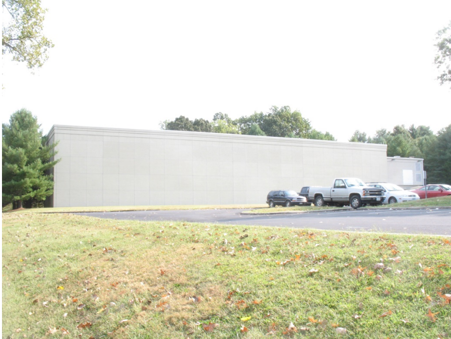
View of Existing Building from Fontana Food Center
