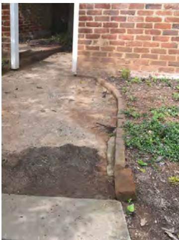
Garden II paving, before test
