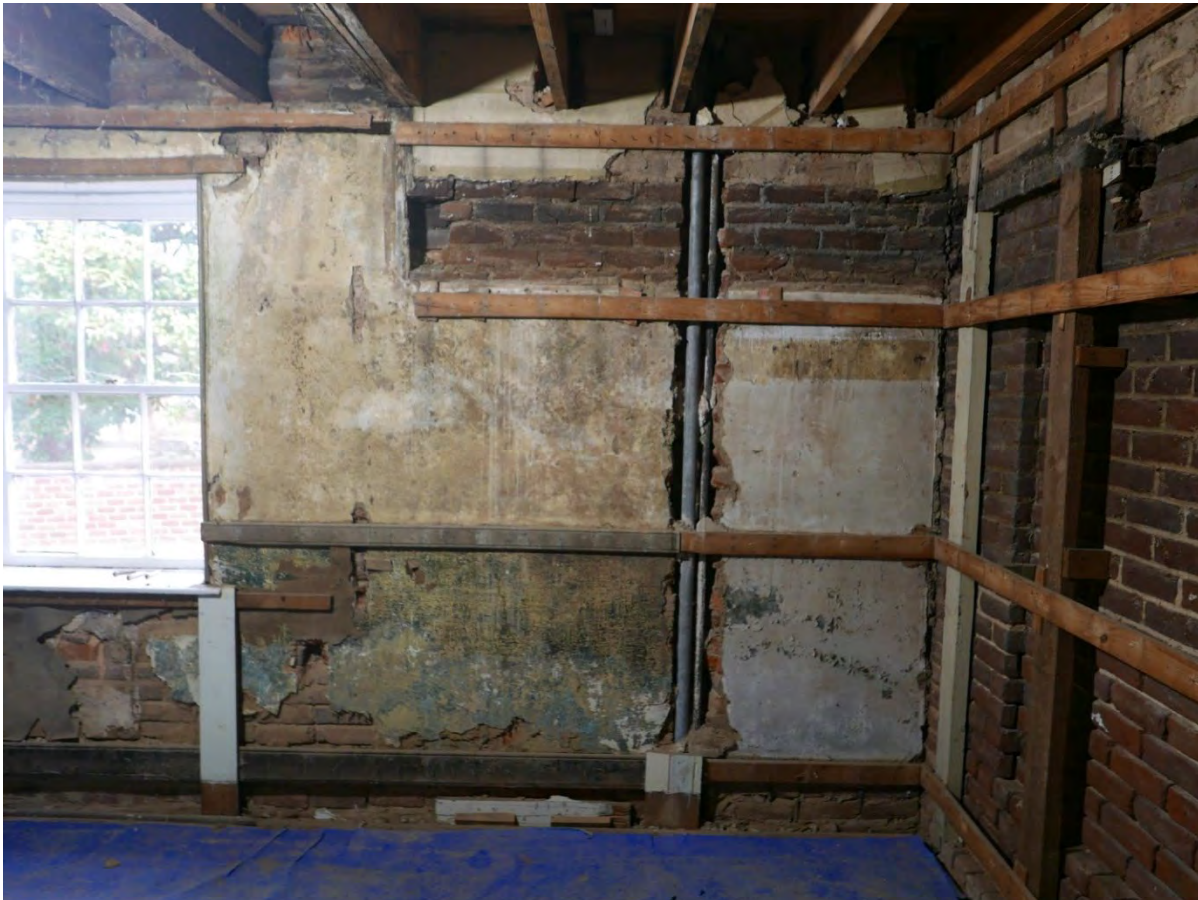
The Mews' original plaster and garden wall shortly after being revealed
