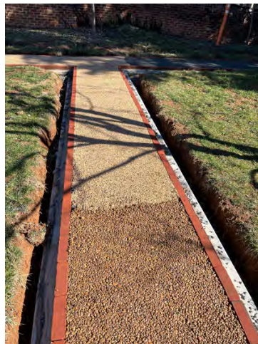
Garden II paving, during test
